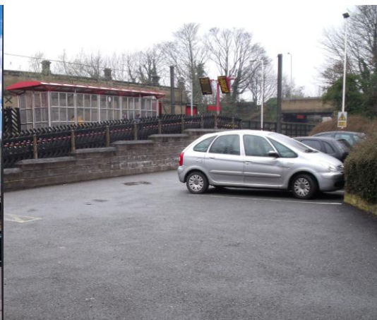
Frizinghall Station Car Park
